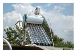
A solar water heater on the roof of a house. The water is in the tank.<sup>5</sup>
