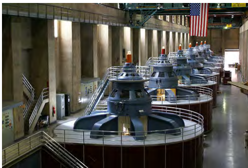
The generators inside the hydroelectric power plant.
