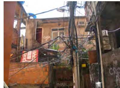
Electricity theft is illegal and also very dangerous due to the insecure connections and fire risks.
