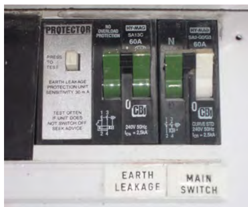
An example of the earth leakage and main switch on a distribution board in a house.
